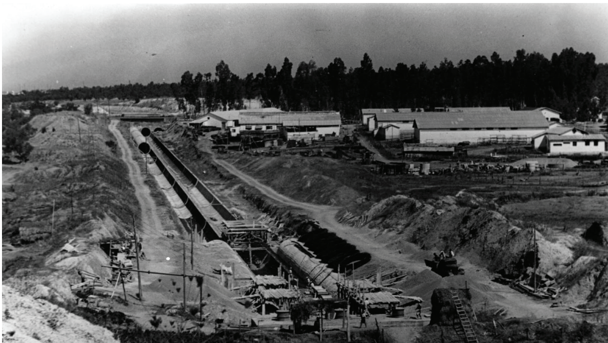
Figure 3: Picture of the penal colony of Los Merinales in Dos Hermanas (Seville, 1945), displaying the construction of an underground water channel, part of the Spanish Inner Colonisation, by war prisoners. Source: Archivo RMHSA-CGT.
