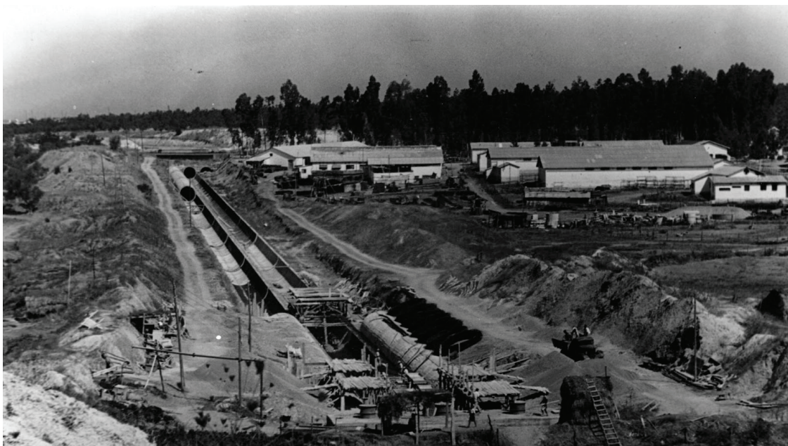
Figure 3: Picture of the penal colony of Los Merinales in Dos Hermanas (Seville, 1945), displaying the construction of an underground water channel, part of the Spanish Inner Colonisation, by war prisoners. Source: Archivo RMHSA-CGT.
